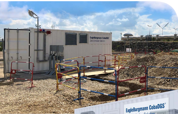
CobaDGS high pressure nitrogen generator and supply system on the operator's site.
